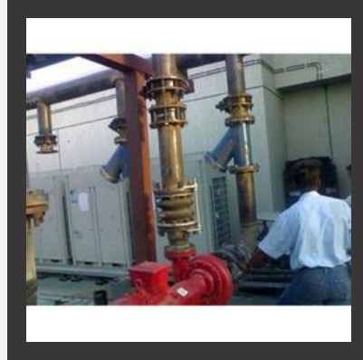
Pump Installation Service
