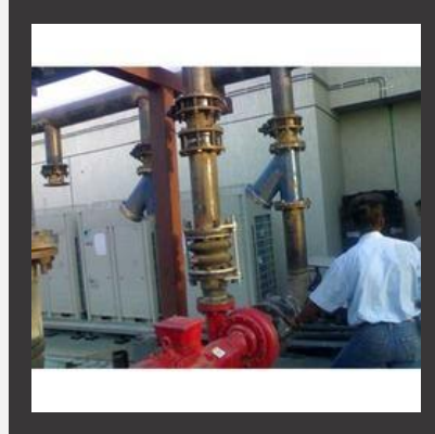
Pump Installation Service
