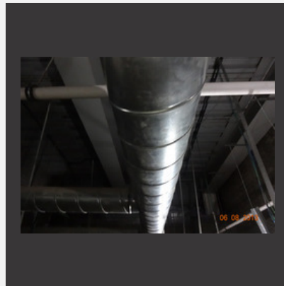
Spiral Duct Installation Service
