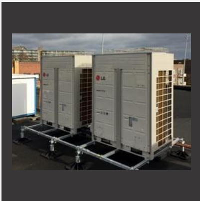
Outdoor Installation Service
